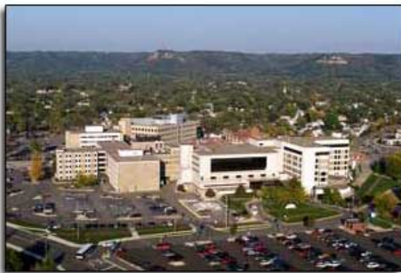
Aerial Photo of Gundersen Lutheran Medical Center, La Crosse
